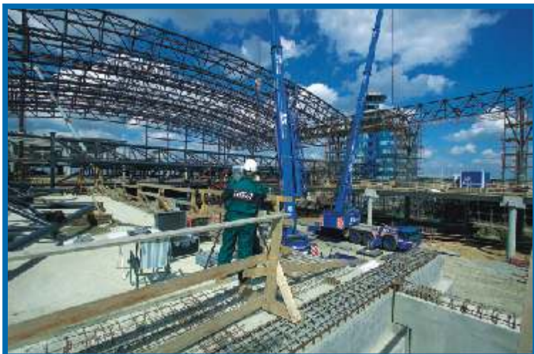
“North” Terminal construction, Prague Ruzyne - Airport
