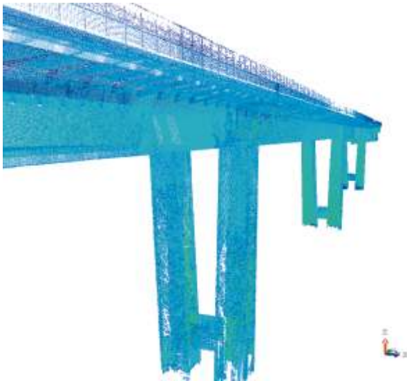
Scan of the Nuselský Bridge and its cells with the metro trackage
