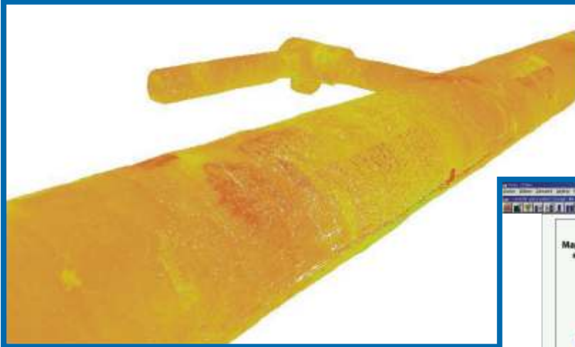
Scan of a metro tunnel line "C", Ládví Prosek
