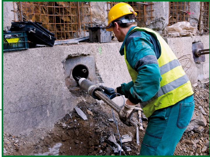
Sensor installation on ground anchor
